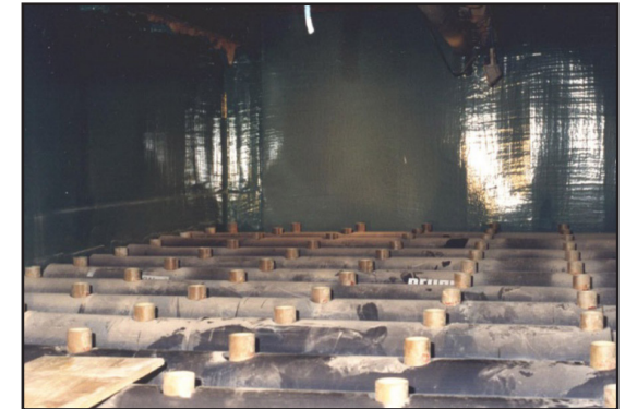
Completed ARC S2 installation in absorber spray zone and smooth surface
