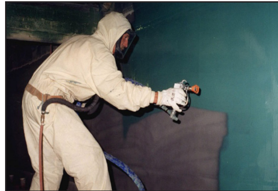
ARC S2 applied using heated plural component airless spray system
